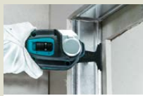
Door opening work
