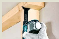
Wood flush cutting
