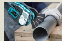
Cutting PVC, FRP pipes
