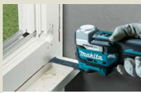
Removal of window frame
